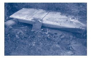
This improperly maintained storm drain does not meet MS4 regulations.
