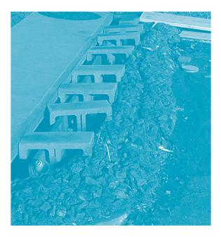
A properly maintained construction site storm drain prevents soil from getting into the drain by utilizing physical barriers. This photo also illustrates how this type of drain system prevents trash from getting into the drain.
