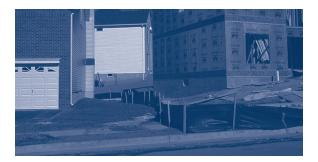
This is a good example of the proper use of silt fencing which acts as a barrier between the property being developed and the adjacent property. Also, it acts as a barrier to prevent runoff of soil and materials onto the street and eventually into waterways.
