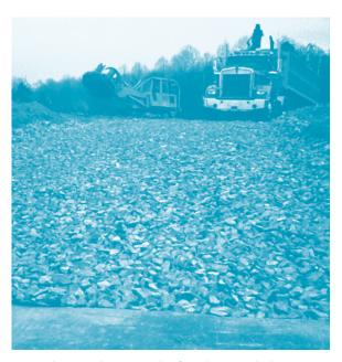
Large, heavy rocks prevent dirt from being tracked onto streets in this properly maintained construction entrance. Dirt on the streets will eventually end up in storm drains.
